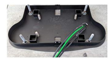
3. Install four more nuts and washers for leveling the system. Set the top of each leveling nut to 44.5 mm (1.75 in) from the top of the bolt.
