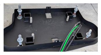
**4.** Feed all three AC conductors and the ground cable, with a maximum size of 35 mm<sup>2</sup> (2 AWG), through the adapter wireway.
