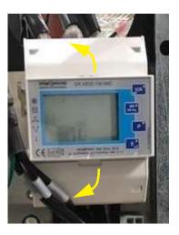
**3.** Use a small slot screwdriver to remove the three small sense wires (A, B, and Gnd) from the top terminals of the meter.
