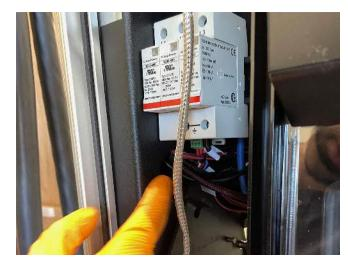
5. From the rear of the station, pull the cable through the grommet on the shelf (from the bottom).
