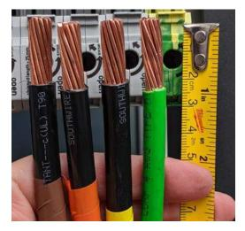
Wires fully inserted into the Wago terminals, with no copper visible, and ports showing no orange tabs
