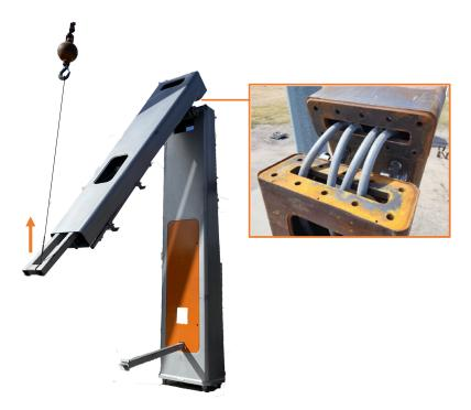
5. Pause when the arm is nearly horizontal and the two connection plates begin to touch. Check the bolt hole alignment between the arm and pole. If required, use a bull pin or iron workers pry bar to align the bolt holes. Then slowly lift the arm until the connection plates mate completely.
