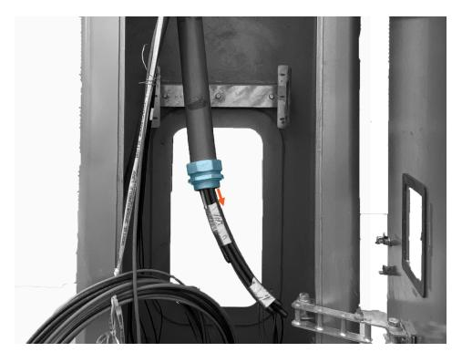
5. At the top of the mast, pull the HV DC wires out the pantograph access opening to fully retract wires into the lower end of the wire conduit. This clears space in the mast for mounting the Power Link 2000.
