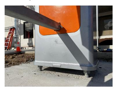
5. Install 2-1/4 inch washer and nut onto each anchor bolt (x4). Tighten to snug tight condition with a 3-1/2 inch socket.
