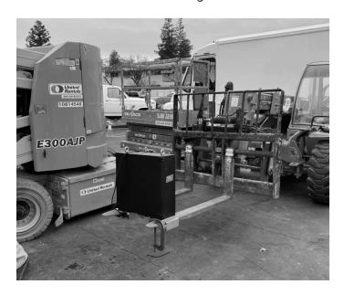
3. Lift and transport the enclosure to the mast. Center the PD Controller in front of the mounting struts.
