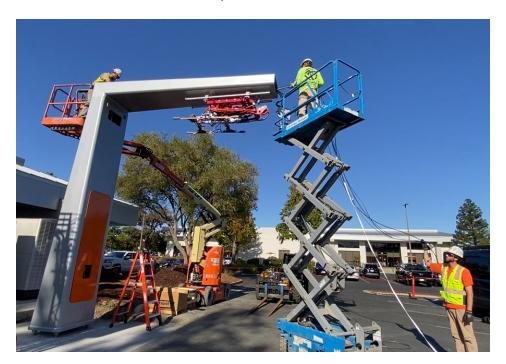
4. Stop when the opposite cable ends reach the front opening of the mast arm. At the top access hatch, secure the cables so they do not slide further down into the pole.
