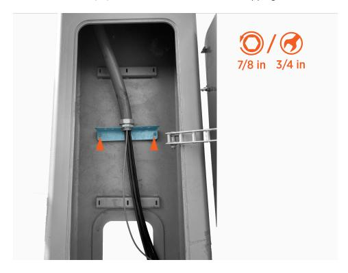
3. Remove the lock nut to release the HV DC conduit from the shipping bracket. Slide the nut and shipping bracket off the HV DC conduit and wires.
