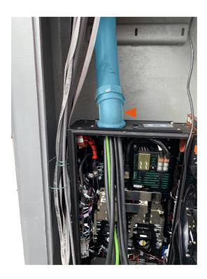
3. Use 3-1/2 in strut pipe strap (contractor-supplied) to secure the HV DC conduit to the strut channel.
