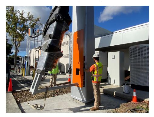
7. Apply Turn of Nut technique to torque anchor bolt top nuts (x4). Use 3-1/2 inch strike wrench.
