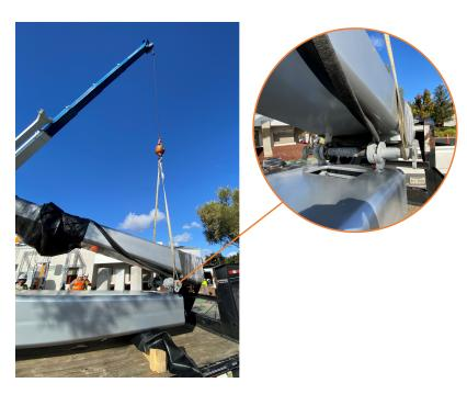
3. Gradually lift and position the mast over and above the anchor bolts.
