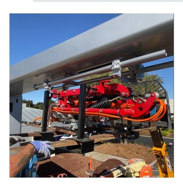
3. Slide each front rail clamps to align its mounting support with a pantograph mounting support. At each mounting point, fasten the supports together with  $5/8 \times 2$  in hex bolt, 5/8 in flat washer, 5/8 in lock washer, and 5/8 in hex nut. Hand tighten.
