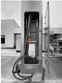
6. Install the Power Link 2000 mounting base using 1/2 in bolt, 1/2 in washer, and 1/2 in nut (x6 each). Ensure the base is level.
